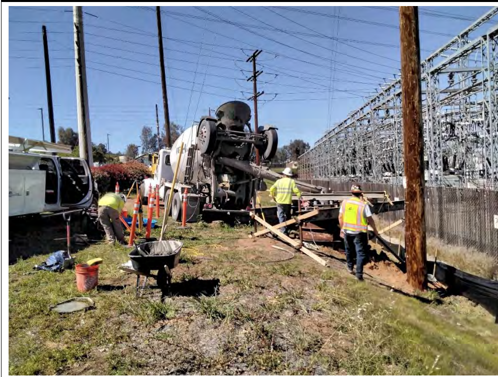
Photograph 7: March 01, 2022. Crews pouring concrete foundation at location 125. Facing: West.
